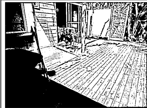
Unit 3. No access under deck.
