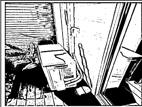
Air conditioning unit overflow discharging against the building
